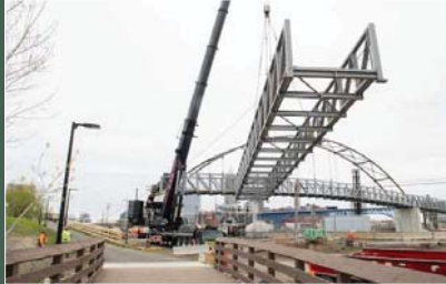
Wendy Park Bridge
