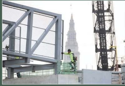
Wendy Park Bridge
